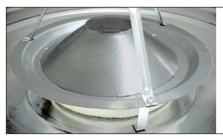
STEP 7: Align outer holes on reflector pan to holes on the reflector pan mounting brackets which have been attached to the canopy.
